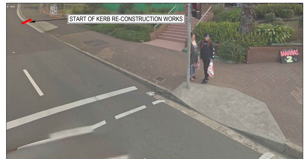
DIAGRAM - MC03 KERB RE-CONSTRUCTION
